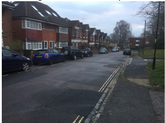
Looking east on Richmond Gardens
